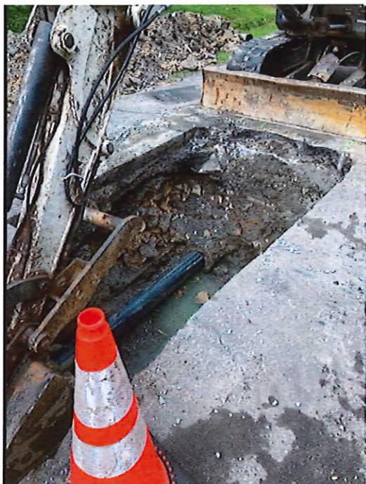
Sliplining new sewer pipe
