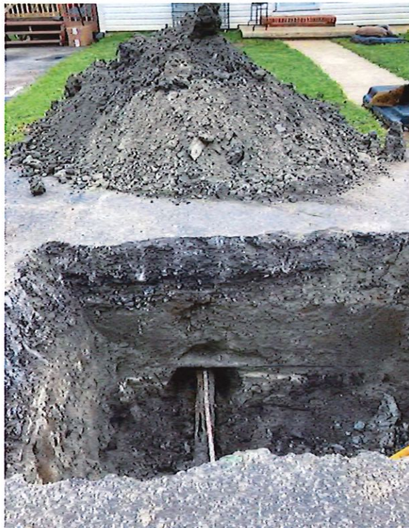
Unearthing deteriorated/aged sewer line for rehabilitation
