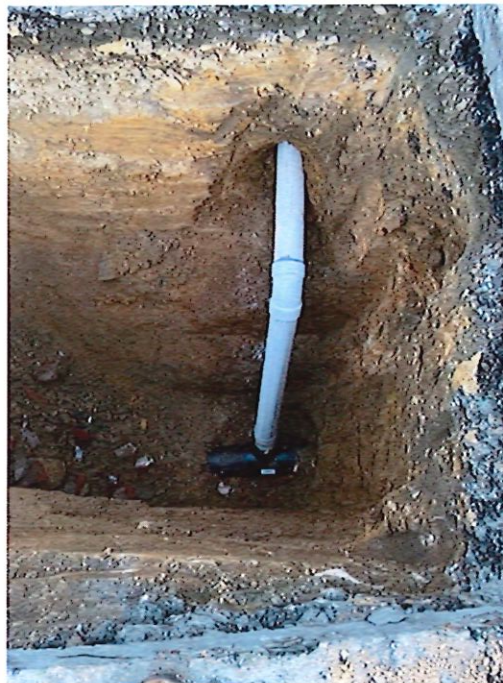
Replacement and connection of new sewer laterals
