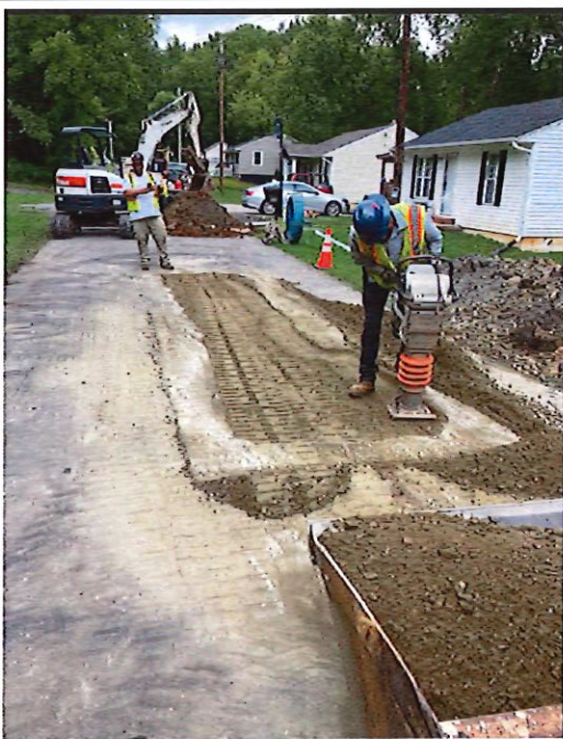
Clean up of construction site and compaction of dirt in preparation for asphalt repair
